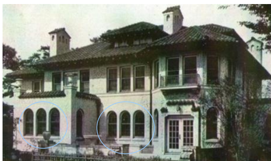
Figure 36. Asabuki Residence (adapted from Vories & Company Architects, 1937)
